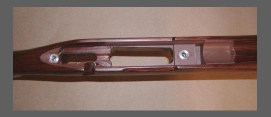
Over time most stocks will crush under the pressure of the trigger guard screws. When this occurs that portion of the stock immediately around the screw will compress much more than the area of the stock in the middle of the action.
